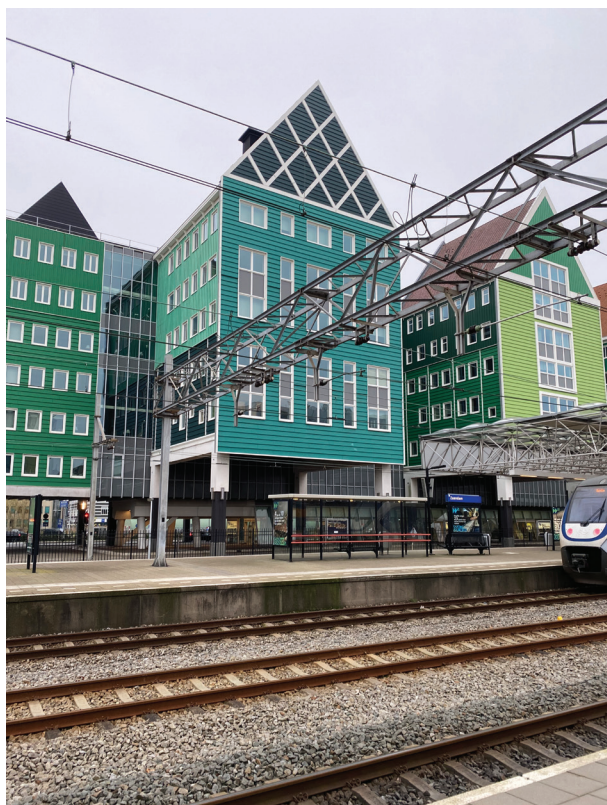
Figure 4. Zaanstad City Hall next to the railway.
